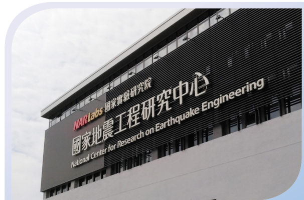
Facade of the NCREE Southern Taiwan Experimental Facility
