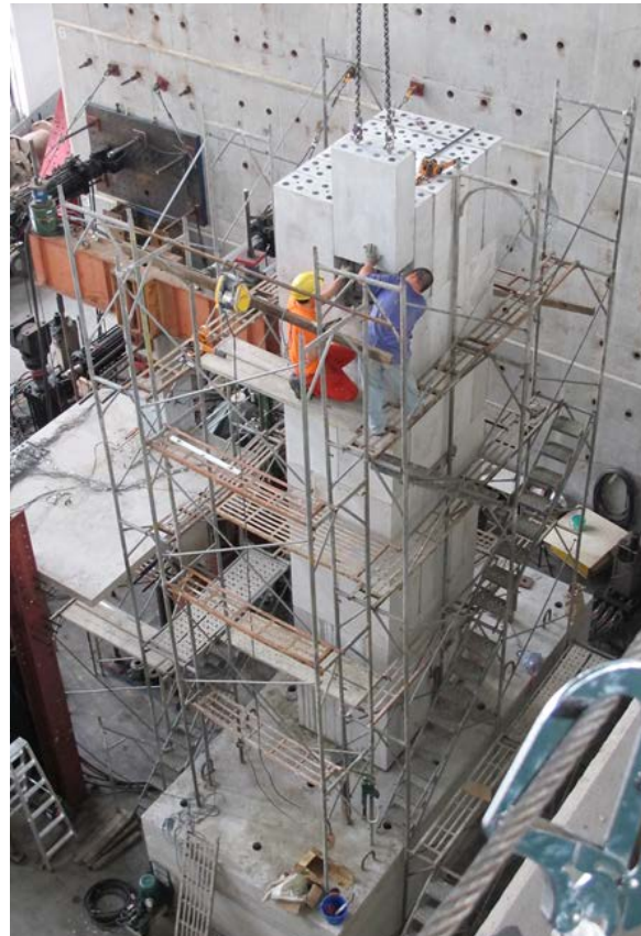
Assembly of pre-cast bridge piers using new biomimetic building blocks
