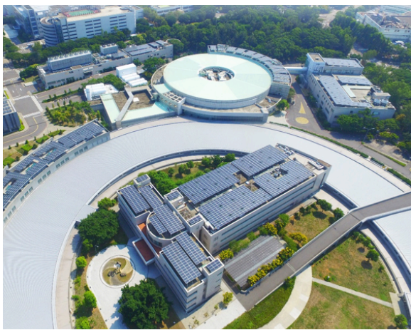
The Synchrotron Radiation Research Center has installed solar panels on the roofs of its buildings; in addition to generating power, this has also beautified the roofs and saved air conditioning costs by blocking sunlight.
